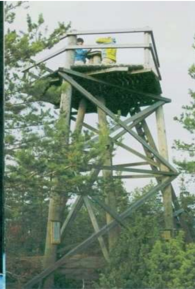
Triangulation tower ("ground reference point") in the Shuve Chain, a member on UNESCO's World Heritage List
